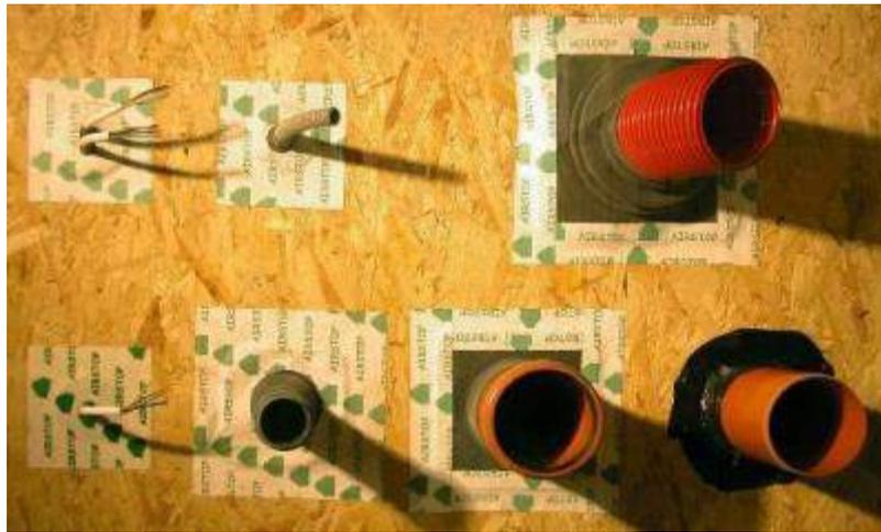
Fig. 2. Perforation sealing
